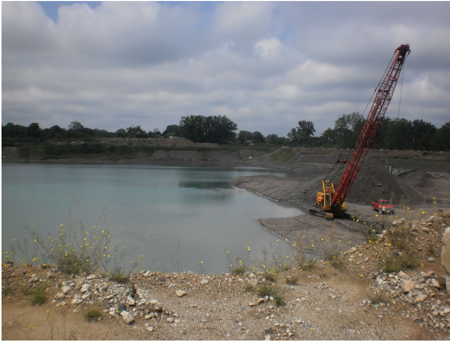
Example of dragline operating at below water pit
